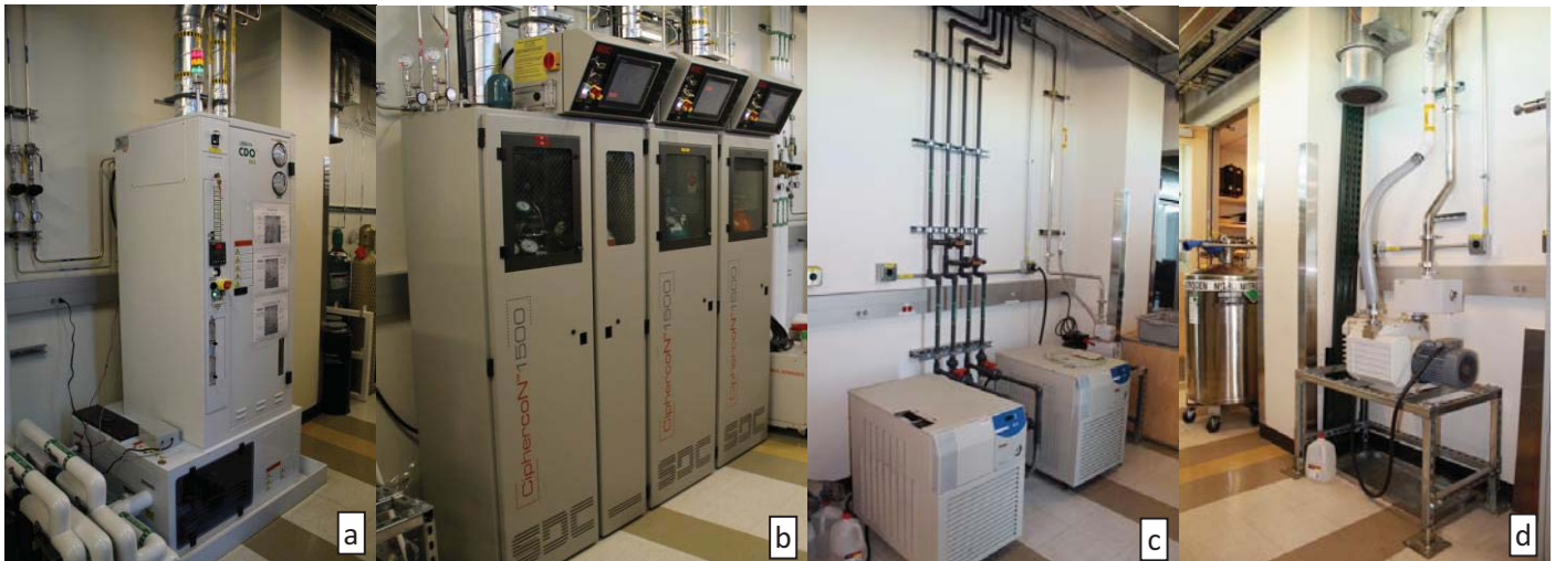
Figure 28: a: burn box; b: safety gas cabinets; a: Recirculating water chiller; b: DUO 65M primary pump, roughing all the turbo pumps of the different systems installed in the lab
